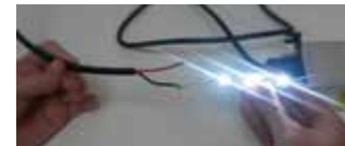
It is an instant way of telling you your transformer is working.
