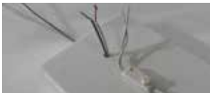
Circuits left open for series wiring onsite.
