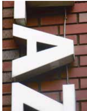
The image shows visible wire between series wired letters.
